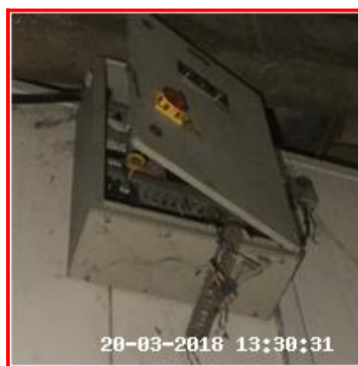
7.13.1 Side Electrical Box - Loose Wires And Cobwebs
