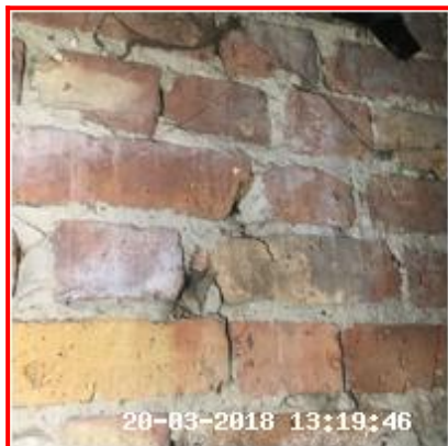
7.5.2 Brick Areas - Pointing Chipped, Bricks Chipped
