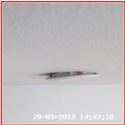
3.3.1 X2 Fitting Not Secure
