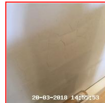
3.4.2 Cracking Behind Fireplace
