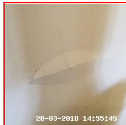
3.4.2 Cracking Behind Fireplace
