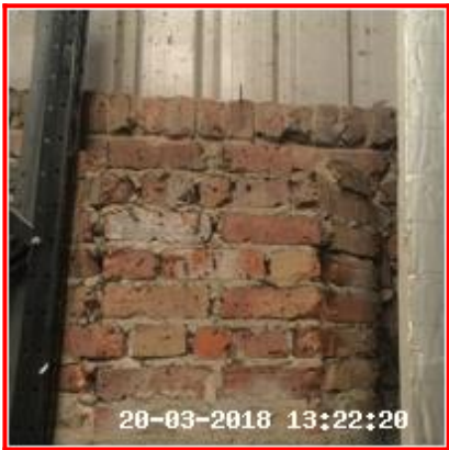
7.5.1 Pointing Chipped, Bricks Chipped
