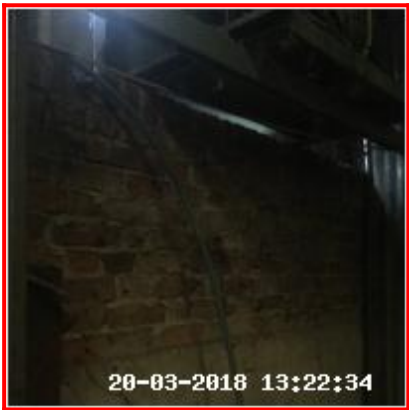
7.5.1 Pointing Chipped, Bricks Chipped
