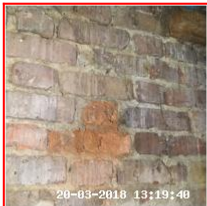
7.5.2 Brick Areas - Pointing Chipped, Bricks Chipped
