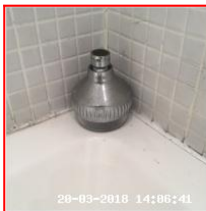
4.9.1 Shower Head Removed, End Taped Up 4.9.1 Shower Head Removed, End Taped Up
