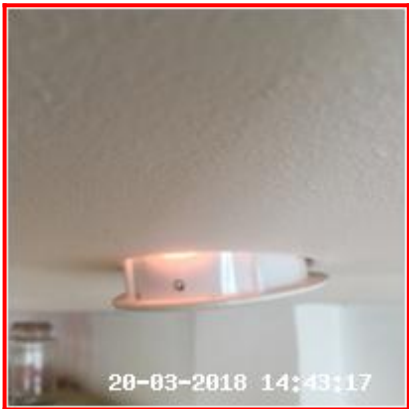
3.3.1 X2 Fitting Not Secure
