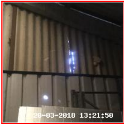
7.5.1 Holes To RHS Cladding
