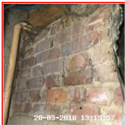
7.5.2 Brick Areas - Pointing Chipped, Bricks Chipped
