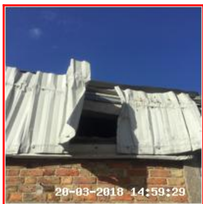
8.1.1 Cladding Damaged Above Disused Toilet
