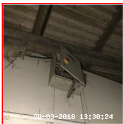
7.13.1 Side Electrical Box - Loose Wires And Cobwebs
