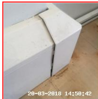
3.4.1 Chipped LHS Of Door Corners Loose To Rear
