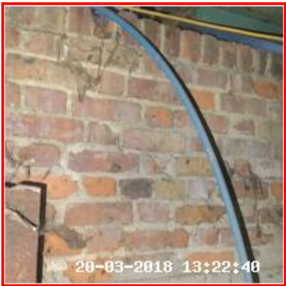
7.5.1 Pointing Chipped, Bricks Chipped
