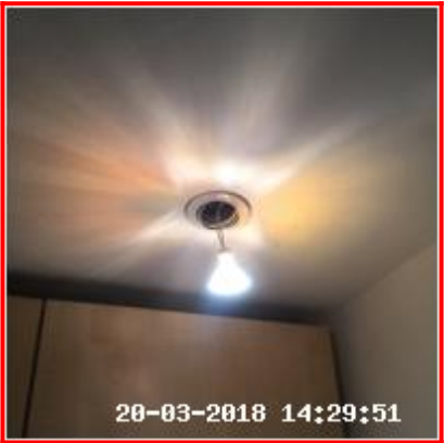
2.3.1 RHS Fitting Not Secure
