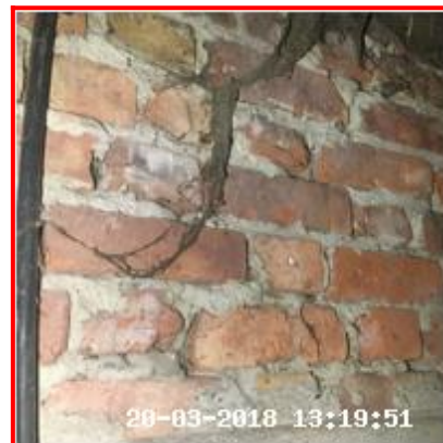
7.5.2 Brick Areas - Pointing Chipped, Bricks Chipped
