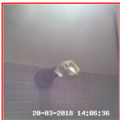
4.9.1 Shower Head Removed, End Taped Up 4.9.1 Shower Head Removed, End Taped Up
