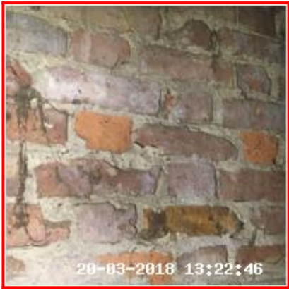
7.5.1 Pointing Chipped, Bricks Chipped
