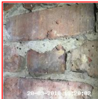
7.5.2 Brick Areas - Pointing Chipped, Bricks Chipped
