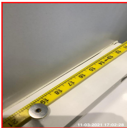
3.10.1 Sealant Damaged To Rear 3.10.1 Sealant Damaged To Rear
