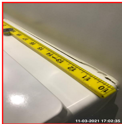
3.10.1 Sealant Damaged To Rear 3.10.1 Sealant Damaged To Rear
