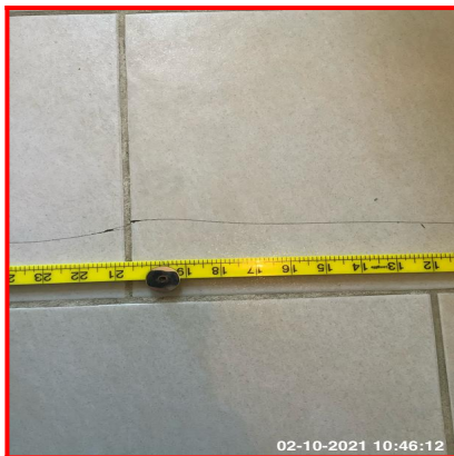
7.8.1 X2 Tiles Cracked By Door
