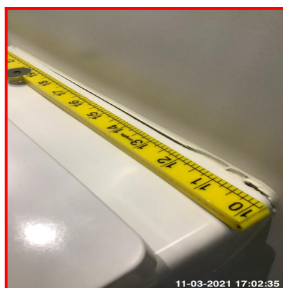
3.1.1 Sealant Damaged To Rear
