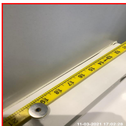
3.1.1 Sealant Damaged To Rear
