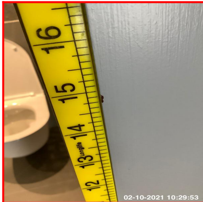
3.1.2 Chip To RHS Edge Above Lock Return
