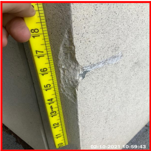
6.2.1 Chip And Scratch To RHS Wall LHS Edge
