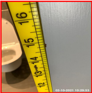
3.1.1 En-Suite (Master Bedroom) Doors / Door Frame Chip To RHS Edge Above Lock Return
