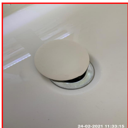
6.1.1 Bathroom Basin Pop Up Plug Not Working. Mechanism Seized In Closed Position
