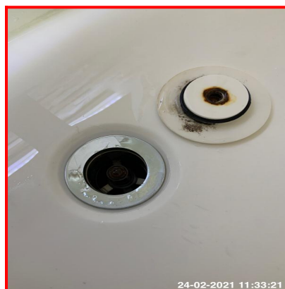
6.1.1 Bathroom Basin Pop Up Plug Not Working. Mechanism Seized In Closed Position
